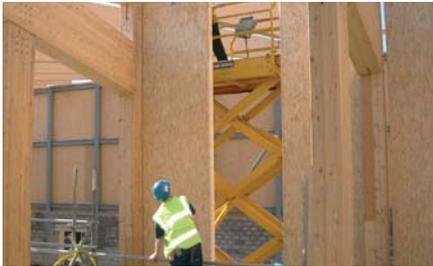
Structural insulated panels (SIPs)
